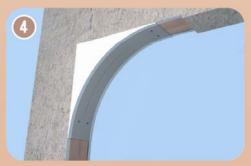
**Tip:** Wetting the back of the drywall strip and carefully curving it by hand are a few
