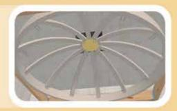
If you'll be hanging a heavy chandelier from the apex of your dome, nail or screw the dome tie through your drywall ceiling into the joists/trusses.
