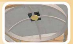
Install the remaining dome rafters by first butting the 11. square cut ends to the dome tie and then sliding the miter cut ends up the dome ring unit they "snap" into the rafter holsters.
