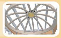
If you'll be hanging a heavy chandelier from the apex of your dome, nail or screw the dome tie into the joists/trusses.
