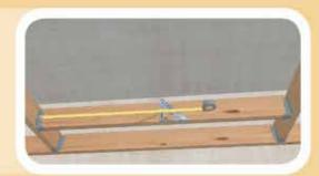
Using a nail gun w/ 16d nails (PROs) or screw gun w/ 3" wood screws (DIYers), fasten each of the 4 dome ring quarter sections with rafter holsters facing up, flush with the bottom or your 5'-0" square box while aligning them to your center lines. If necessary, the dome ring quarter sections can be flexed to meet the center lines.
