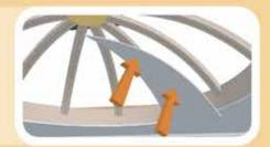
Once the pie-shaped pieces are in place, use a screw gun and drywall screws to fasten in place.
