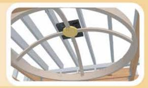
10. Install the remaining dome rafters by first butting the square cut ends to the dome tie and then sliding the miter cut ends up the dome ring unit they "snap" into the rafter holsters.
