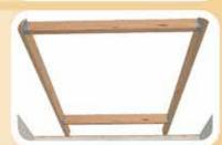
3. Using a tape measure and square, measure and mark center lines on all four sides of your 5'-0" square box (2'-6" or 30" in from each corner).
