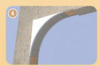
Tip: Wetting the back of the drywall strip and carefully curving it by hand are a few tricks the Pro's use to attach drywall to a curved surface.
